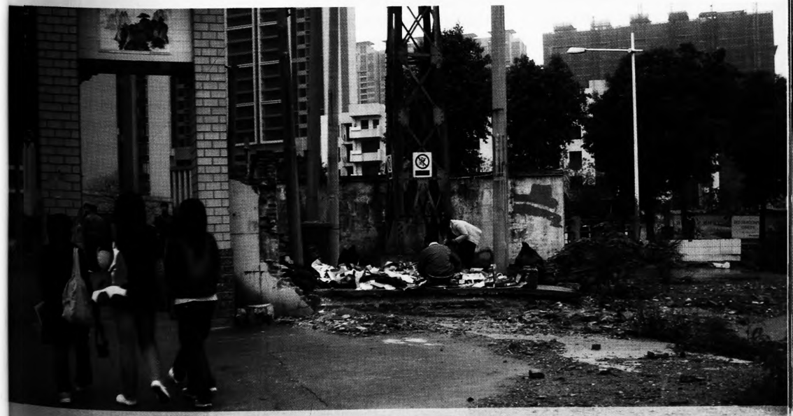
Image 2. Liede: Demolition begins, 2009. Photo by Marco Cenzatti.
